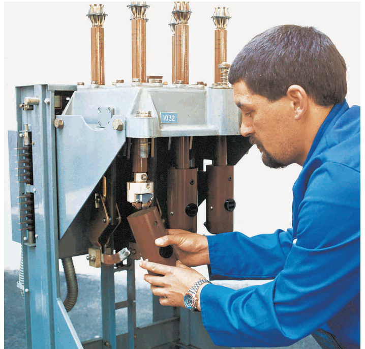
Servicing a 630 amp oil circuit-breaker.
