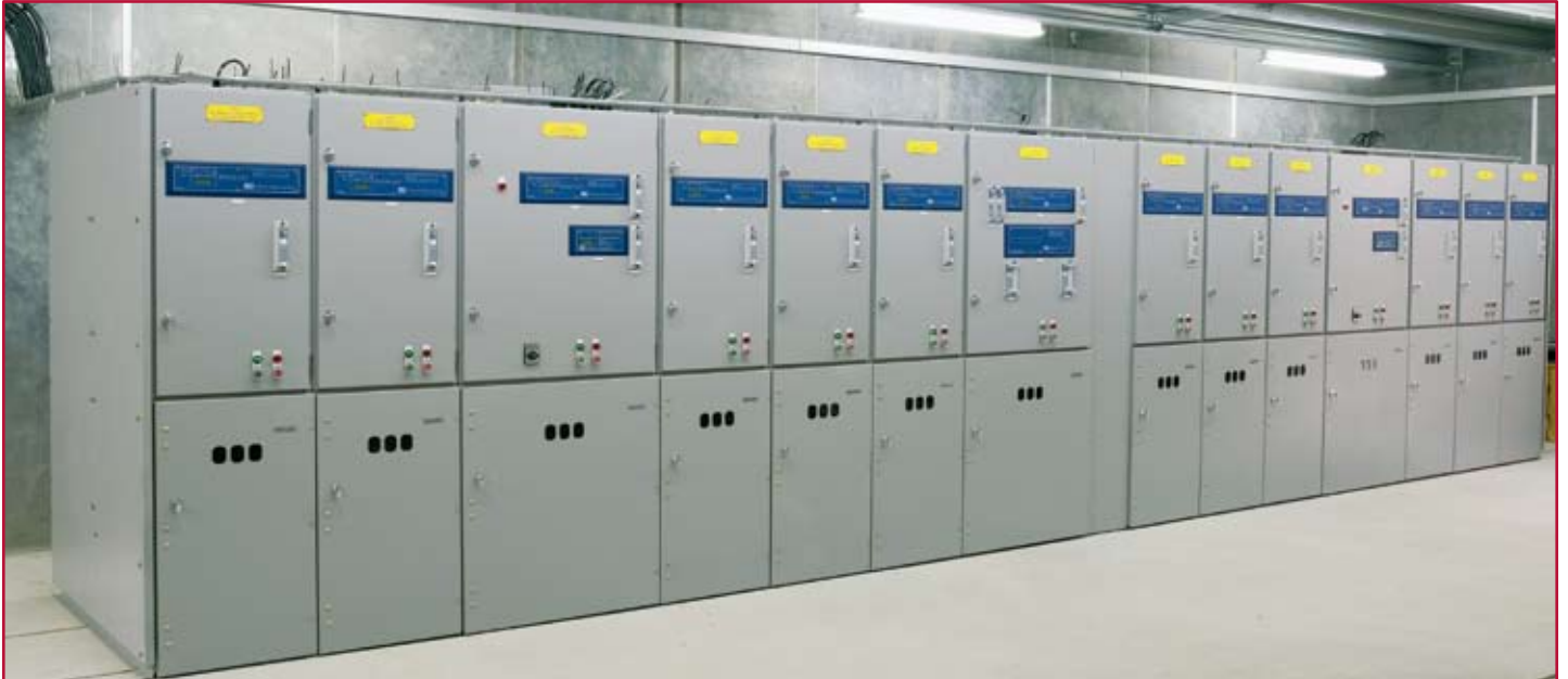
LMVP Switchboard Installation: Powerco – Main St Substation
