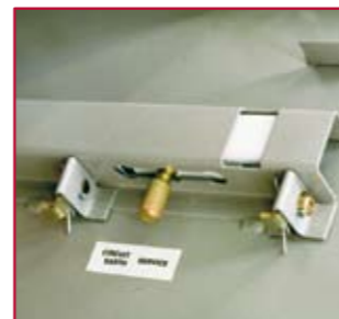
Selector gate mechanism for circuit-breaker
