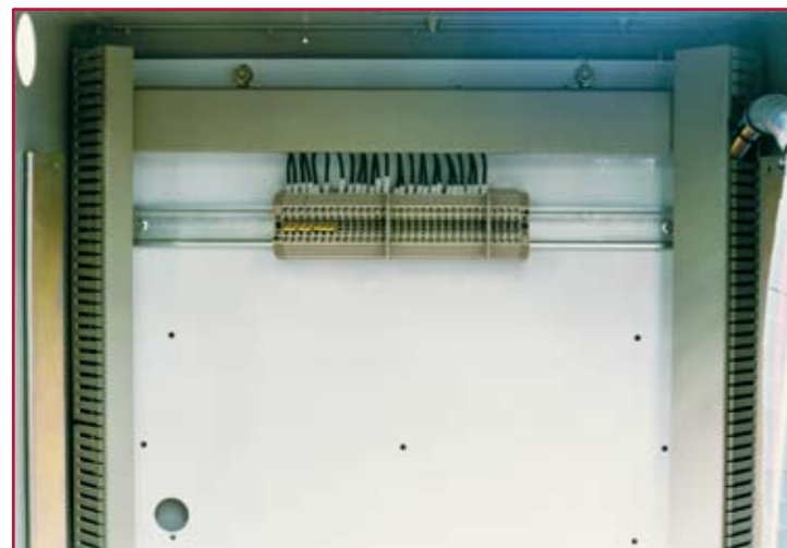
Control & Indication Cable Terminal Blocks
